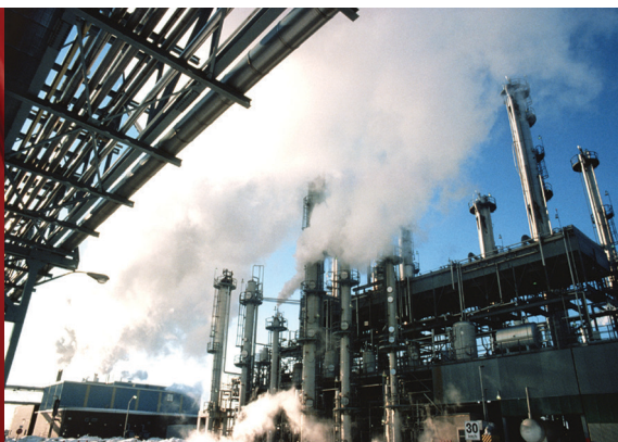
Instrumentation and Automated Pneumatic Controls
